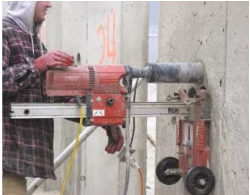
Figure 6: Cores were taken from each wall.
