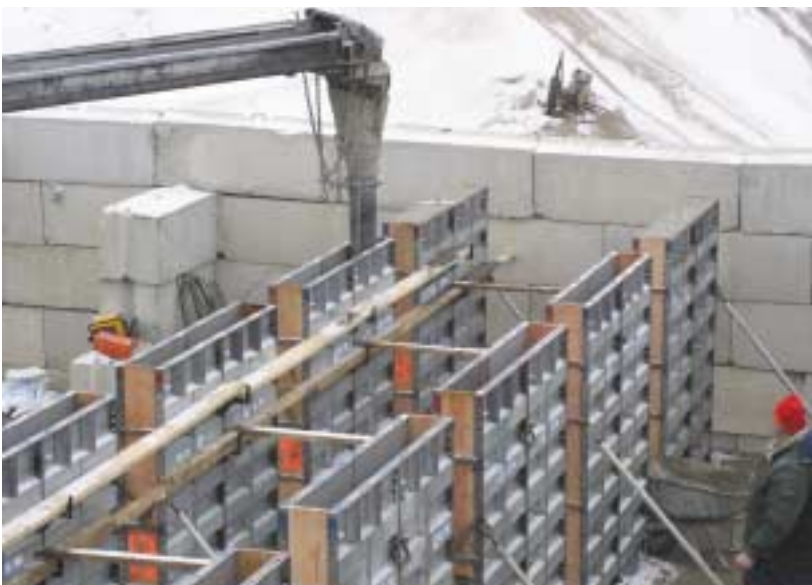
Figure 4: Full-scale testing of the walls.
