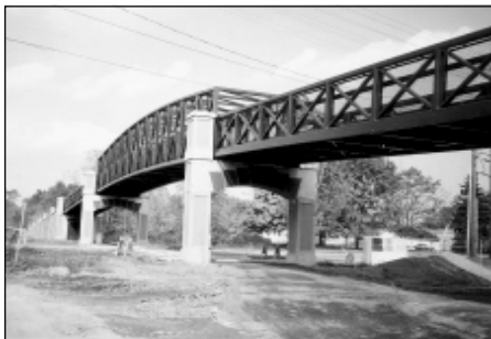
The completed structure has a reinforced concrete deck on corrugated steel deck forms.
